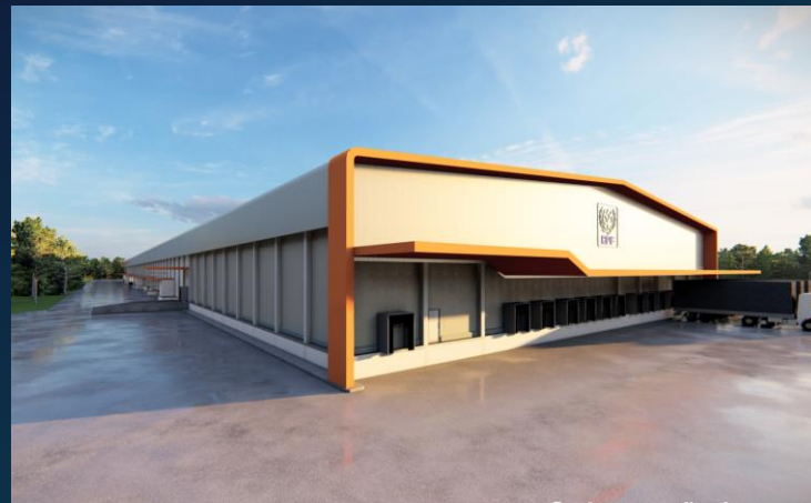
Lopburi Swine Slaughtering and Processing Plant
